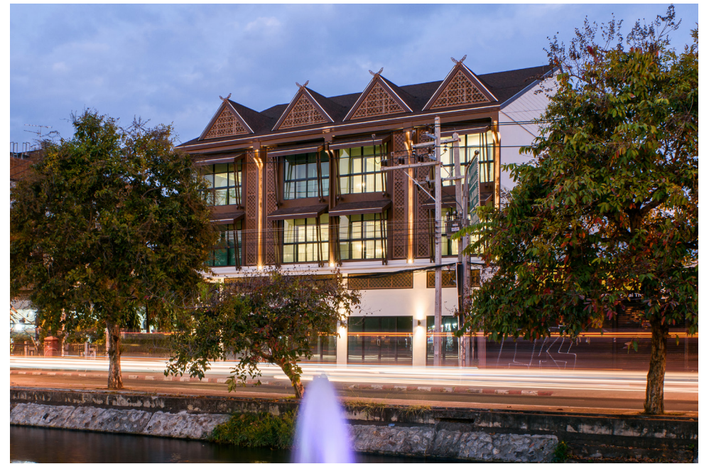
↑ the building after extensive renovations
